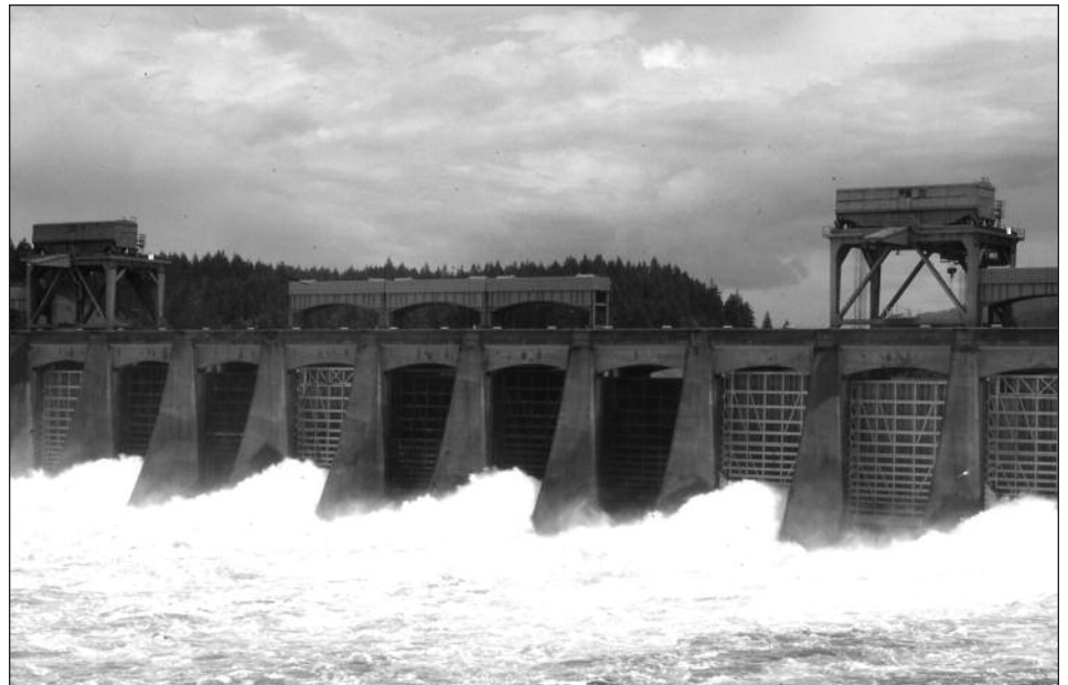
Increasing spill at the dams on the Columbia and Snake rivers hydro system has been shown to improve juvenile salmon and steelhead survival. Photo by Jim Yuskavitch
